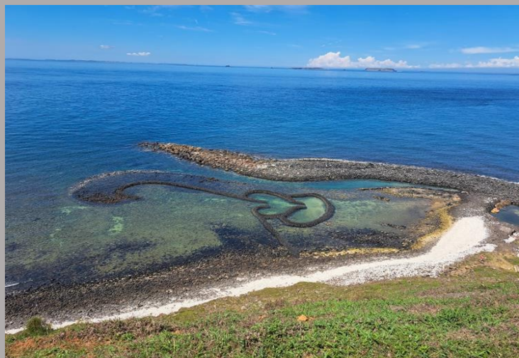
Photo: The famous twin hearts stone weir of Chimei. It is a clever adaptation of local tidal conditions to catch fishes. The former name of Penghu islands was “Pescadores” which means fishermen in Portuguese.
