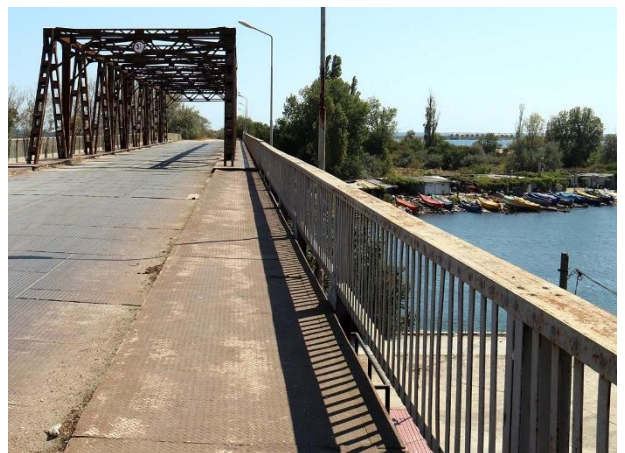
Bridge to Insula Mangalia, Romania (photo by Ilan Kelman)
