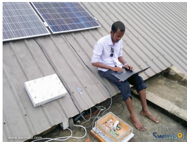
Swimsol's employee Akram Ali carrying out maintenance work on a rooftop
